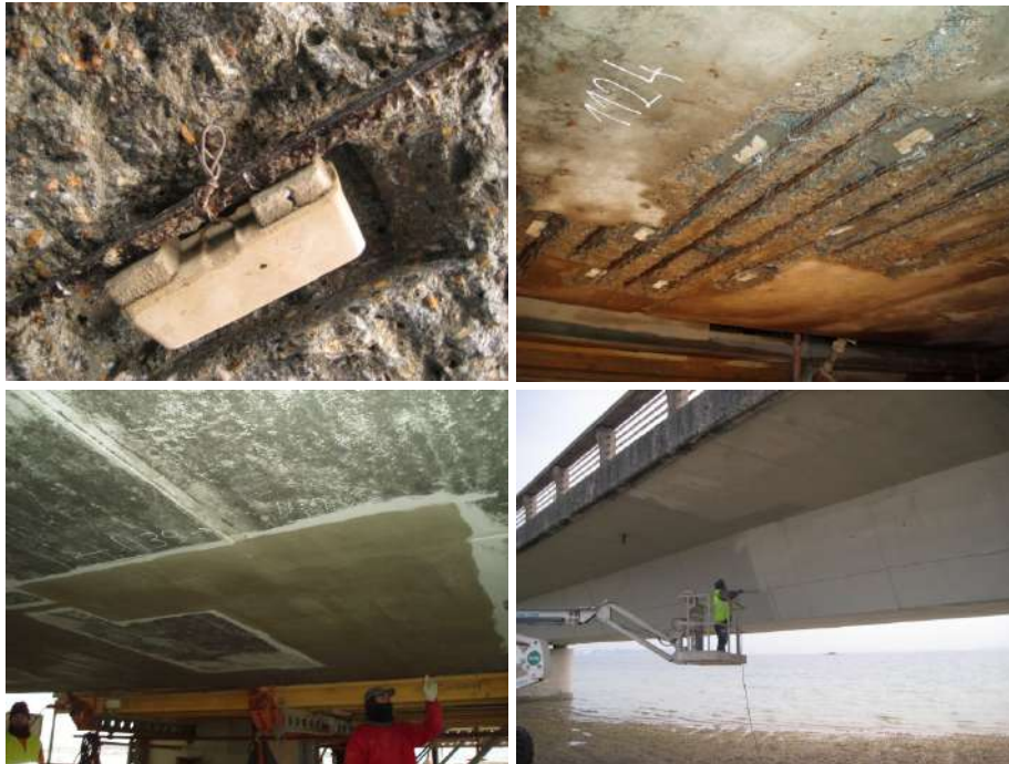
Figure 6. Details of the repairing procedure (sacrifice anodes, application of mortar patches and final painting)
