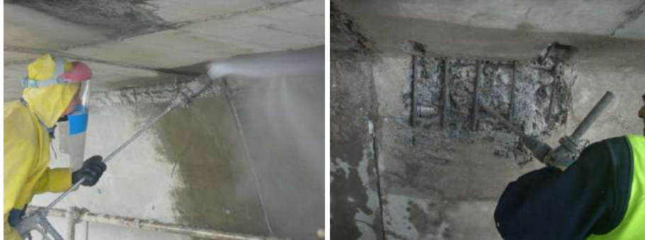
Figure 4. Techniques of demolition of damaged areas of the deck.
