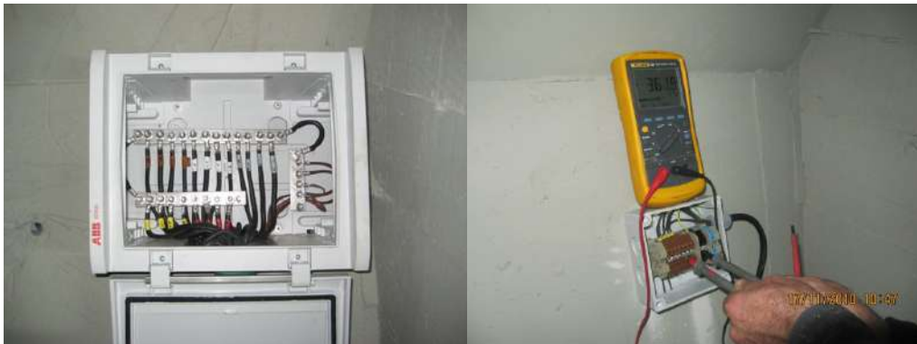
Figure 9. Detail of a connection box and the procedure of measurement of the voltage
